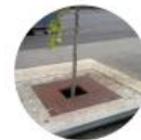
Stormwater tree trench
